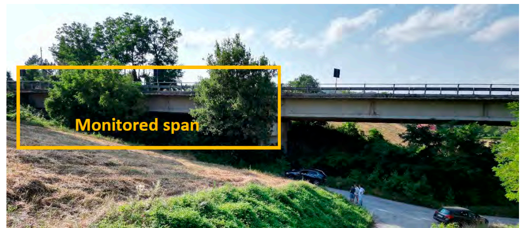
Figure 8. Lateral view of the case study bridge on the day of testing.
