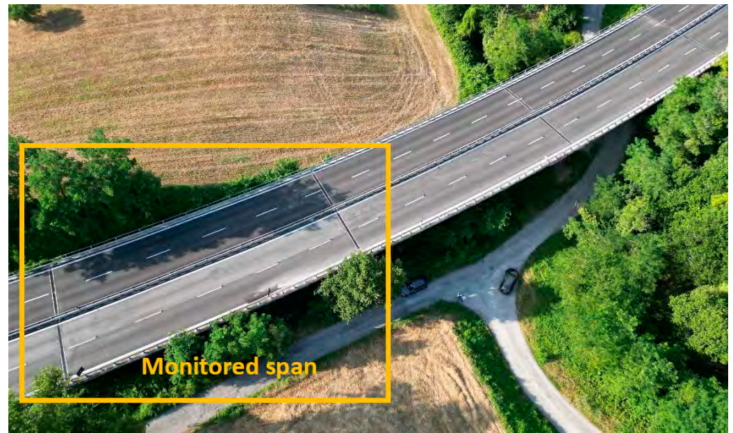
Figure 7. Aerial view of the case study bridge on the day of testing.
