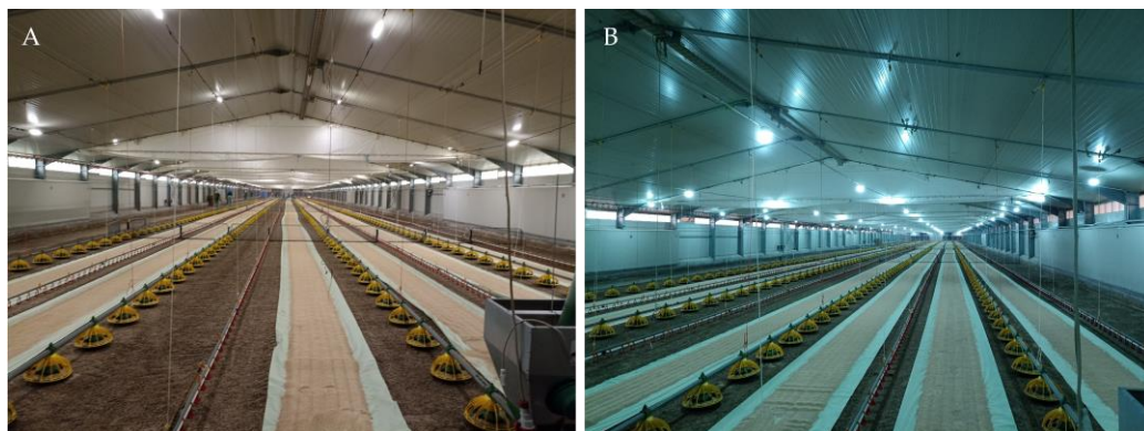
Figure 1. Poultry houses used in this trial. (A). Poultry house WL, equipped with compact fluorescent white light. (B). Poultry house BSL equipped with broiler-specific light (NatureDynamics System, ONCE by Signify, Philips).
