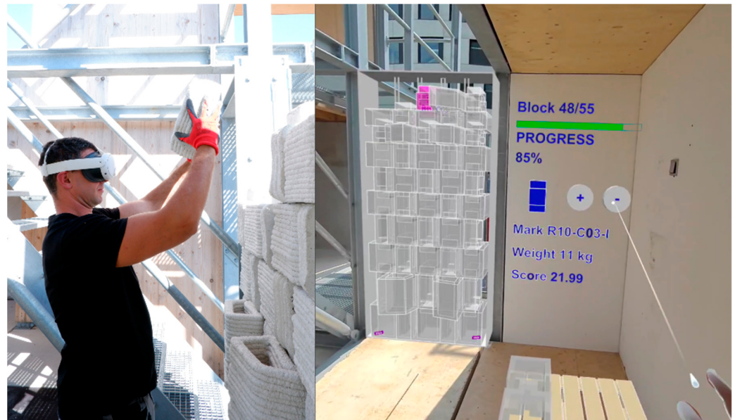
Figure 10. MR-assisted assembly process using a Meta Quest headset (Meta Platforms, Menlo Park, CA, USA) and Fologram (Fologram Pty Ltd., Melbourne, Australia), supporting element positioning, sequencing, and traceability within the digital twin environment.
