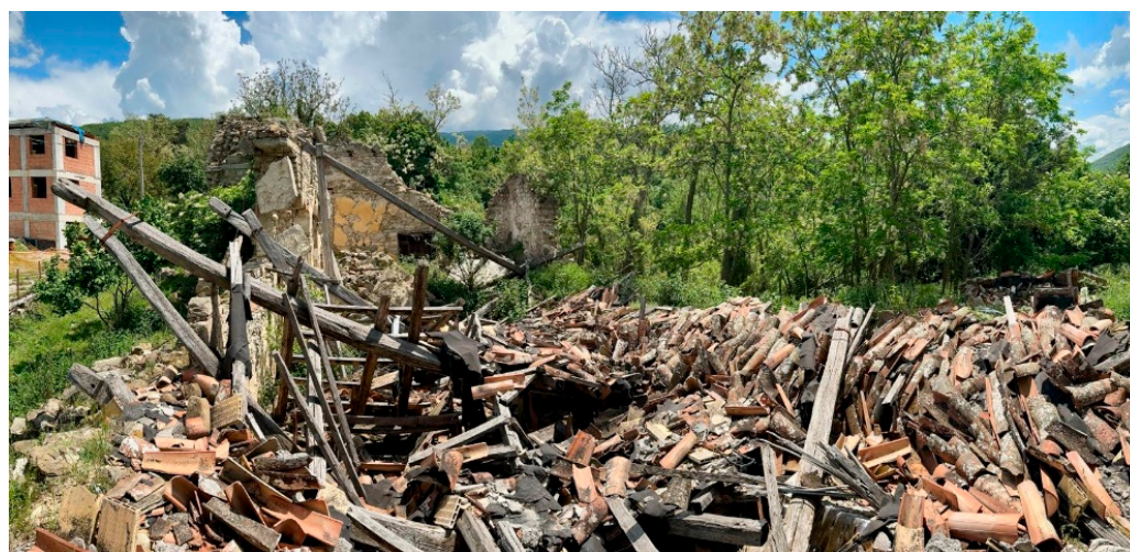
Figure 1. Heterogeneity of materials in a collapsed building following the 2016 Central Italy earthquake (Accumoli, RI), illustrating the mixed and unsegregated nature of seismic rubble that constrains reuse and circular processing.
