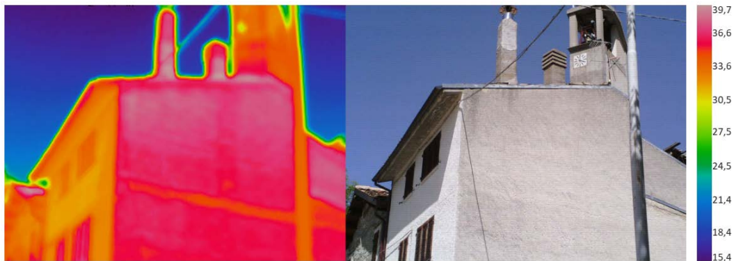
Fig. 6: Example of a thermographic survey
