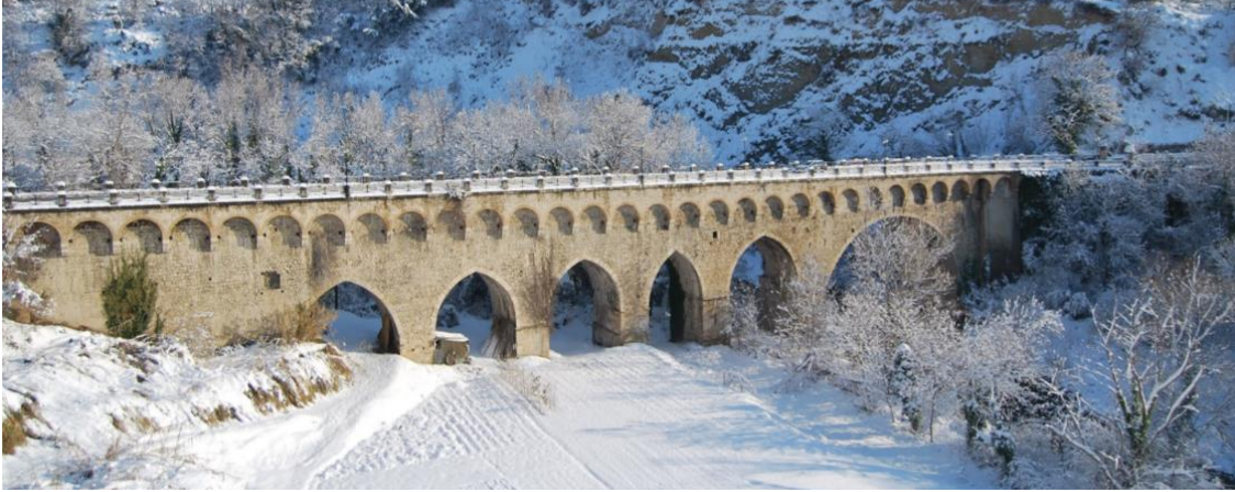
Figure 1: Aerial photogrammetric bridge view.
