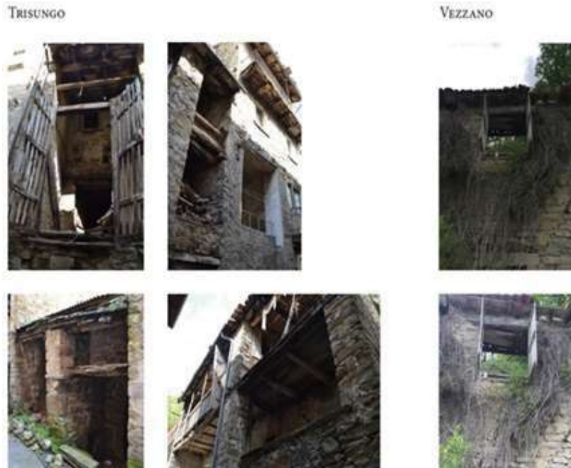
Fig.3.4 Examples of dryers in Arquata del Tronto. (source: authors)
