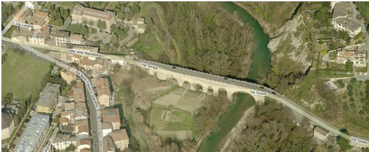
Figure 1: Aerial photogrammetric bridge view.
