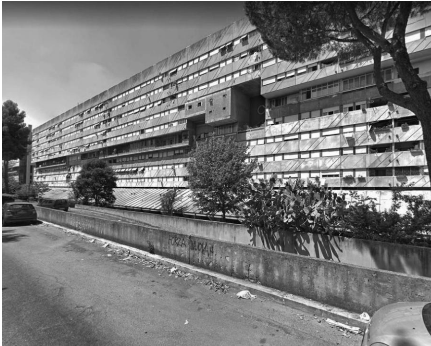
Figure 6 Corviale. Photo from Google Earth.
