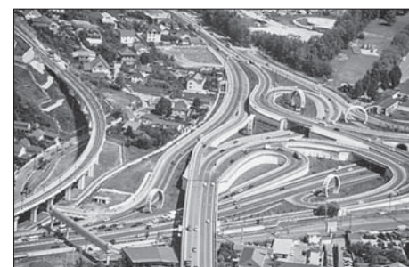
FIG. 12 ONE OF THE NEW MOTORWAY JUNCTION OUTSIDE SOCHI
