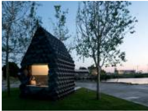
Figure 2.12 3D Printed Urban Cabin 77
