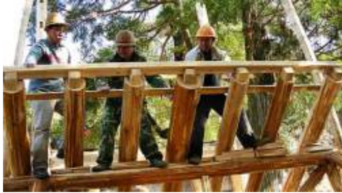
Figure 2.8 Chinese Wooden Arch Bridge 56
