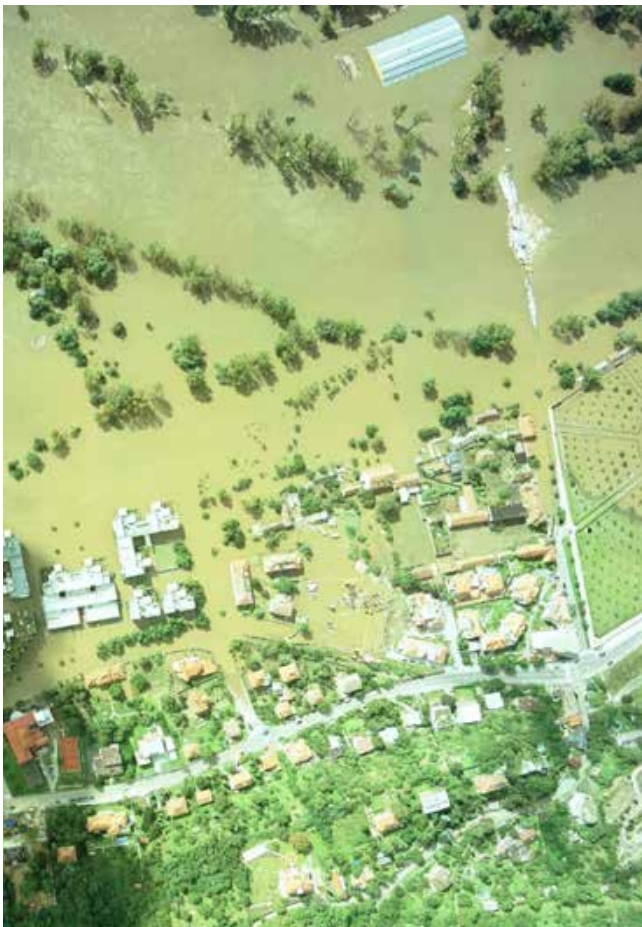
Fig. 4 Comparison of the extent of flooding of the residential area before and after the construction of the flood protective embankment (floods in 2002 and 2013). © Archives of the Troja Municipal District.
