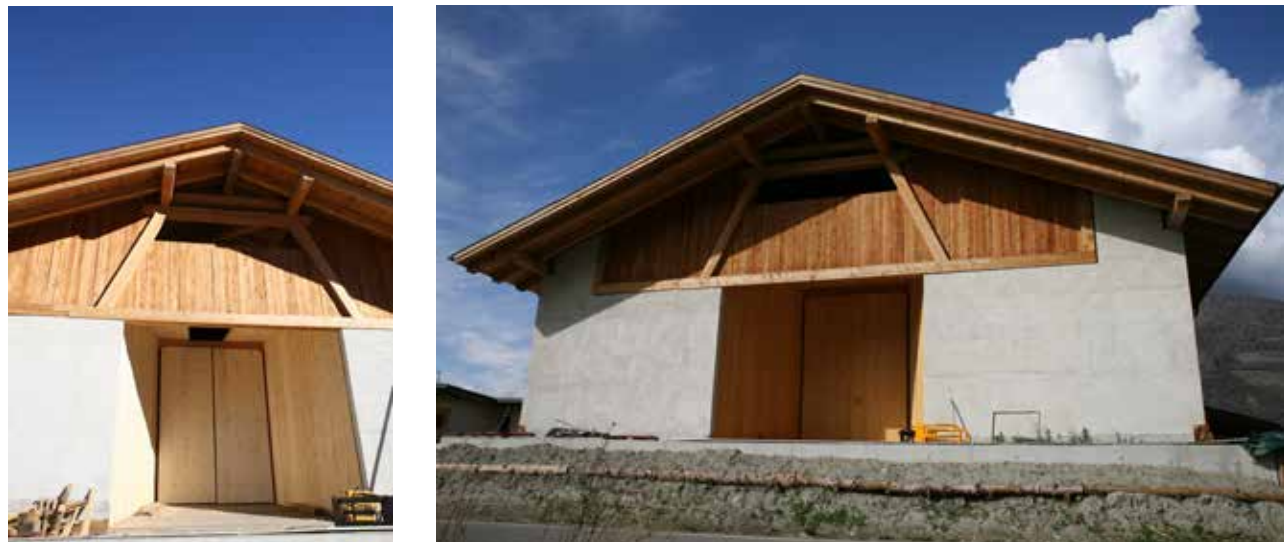
Fig. 1 Entrance area of a new stable and barn building in the form often found in the Vinschgau Valley. Wood species: larch and spruce. Plastering as lime plaster with lime putty as a binding agent. The sand comes from the immediate surroundings and has special colour effects indoors; outdoors it produces a surface typical of the area after (slight) weathering. (Photo: Josef Perger)
