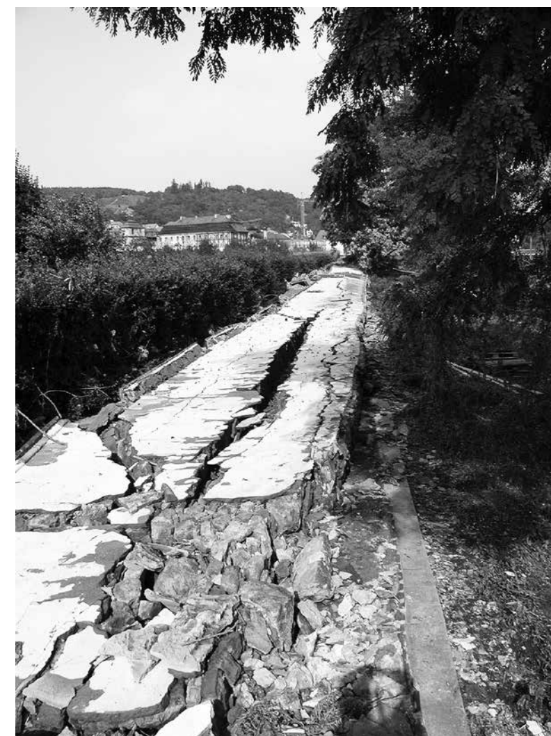
Fig.1 The Collapsed late Baroque stone masonry garden wall in Troja Chateau – Praha 7 (flood 2002). © M.Drdáký
