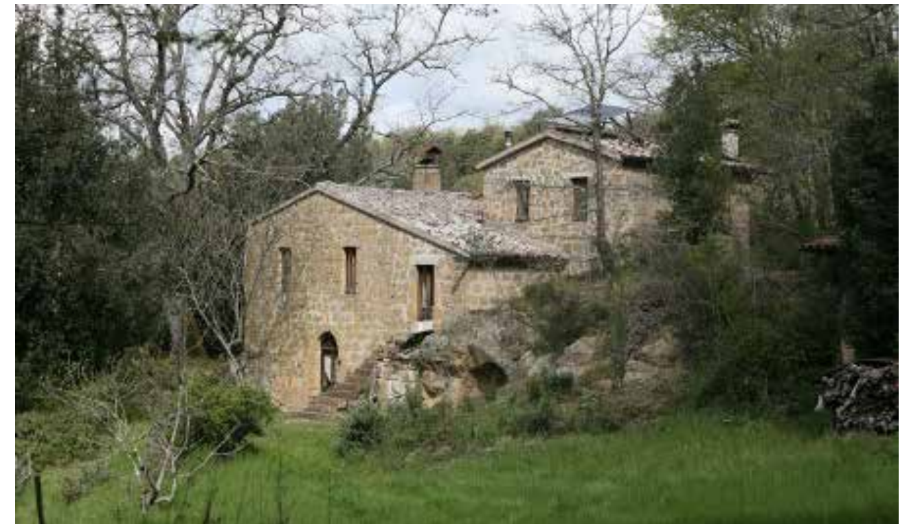
Fig. 2 Extension of a medieval Tosco-Latio building with a 'Stöckel building' (right in the picture). The extension turns the house with 1 room (above the cellar), which was difficult to use, into a house with 3 rooms plus bathroom. Materials: Tuff partly from demolition, partly newly cut and a little travertine. (Photo: Josef Perger)
