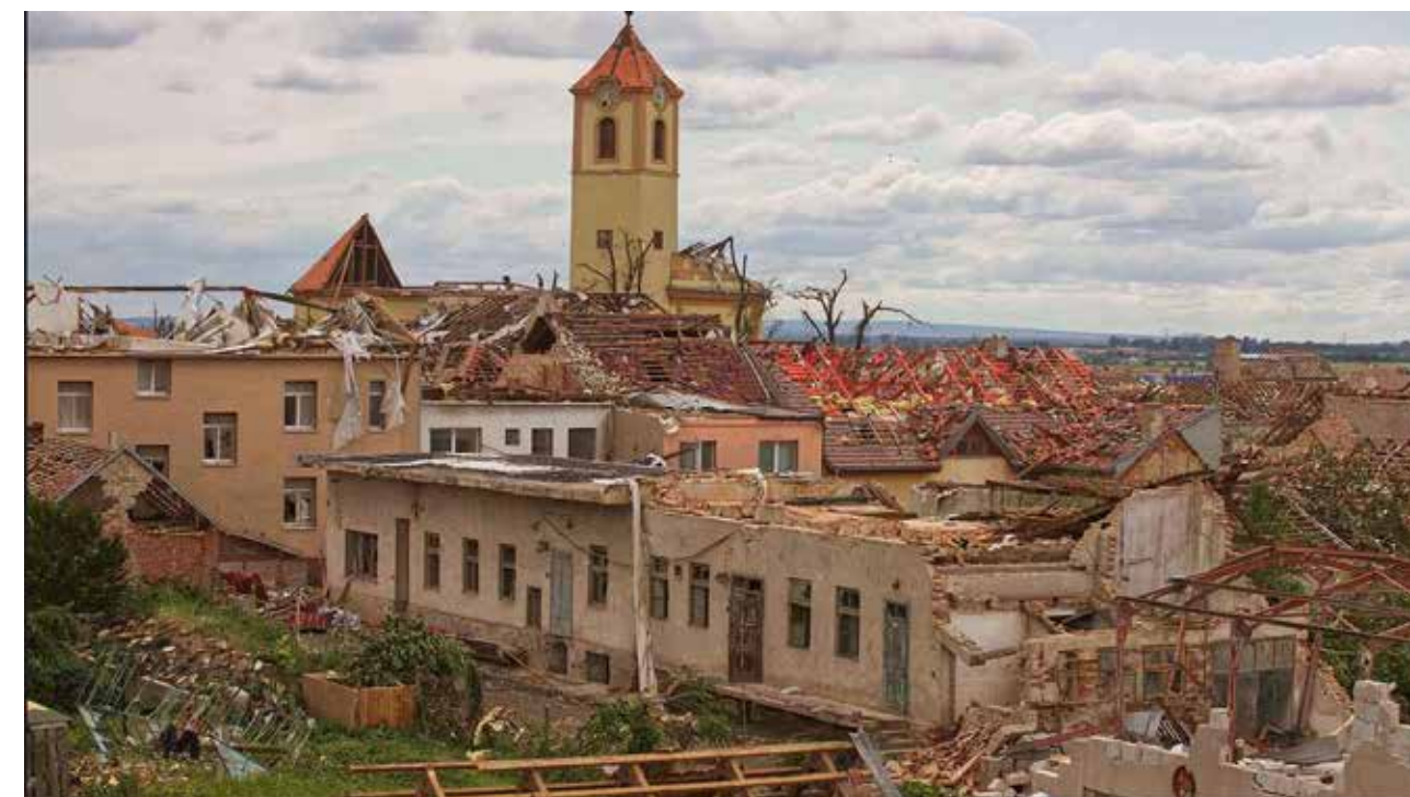
Fig. 4 - A view of a part of the tornado-damaged Moravská Nová Ves with the Church of St. James the Elder in the middle. Source: https://katyd.cirkev.cz/vydani-20210629/z-domova/tornado-nicilo-ale-odkrylo-lidskost_8716?media=desktop
