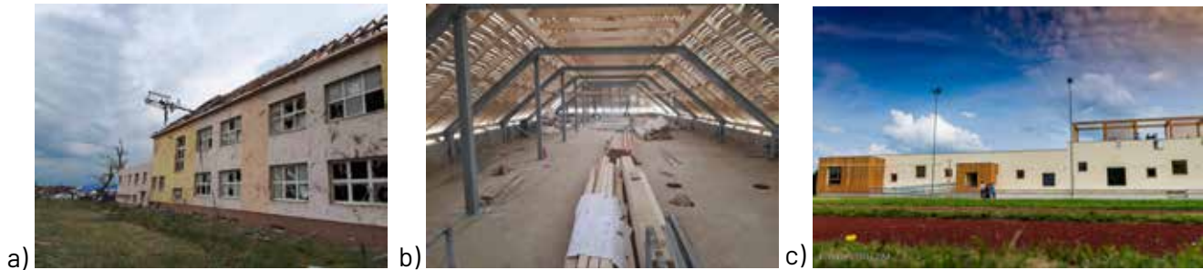
Fig. 7 Elementary school: damage after the hit (a), repaired truss (b), completed extension (c). Source: https://www.mnves.cz/projekty/oprava-budov-po-tornadu-zakladni-skola-2-stupne-mestanka/
