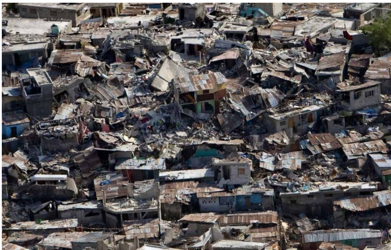
Fig.3 Example of damaged areas of poorly maintained buildings (Haiti).
