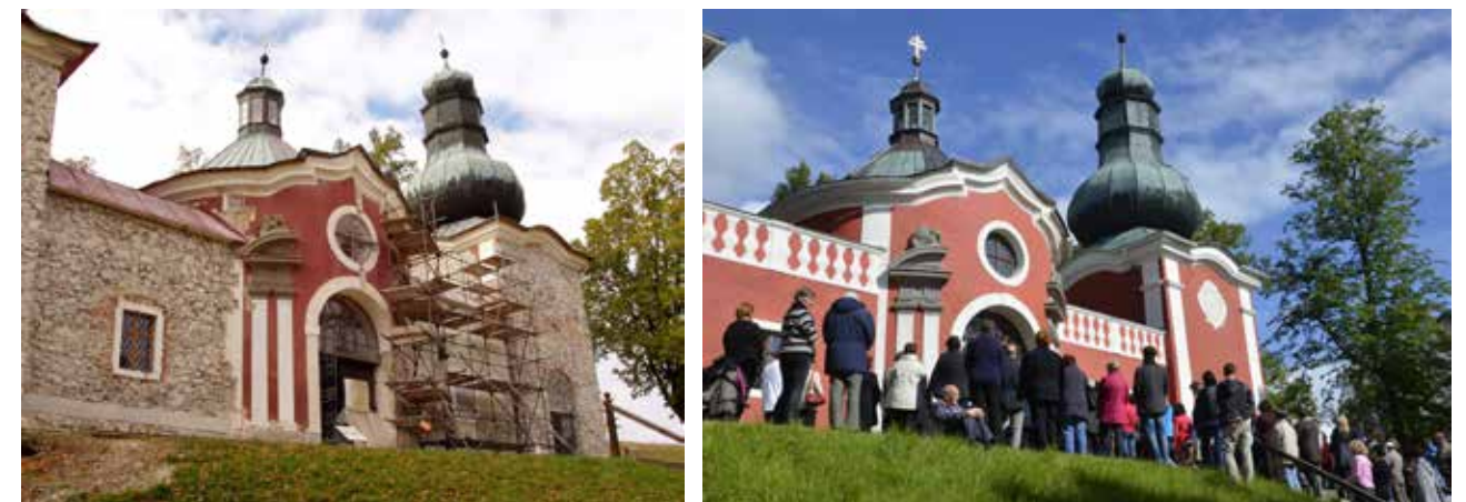
Fig. 11,12 The Lower Church of the Calvary Complex before and after restoration. Archive of Authors.
