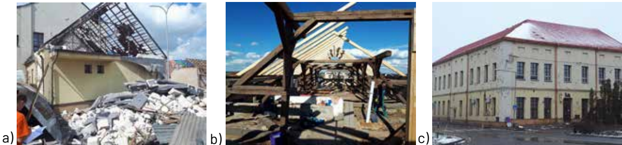
Fig. 9 House No. 117: damage after the hit (a,b), repaired building (c). Source: https://www.mnves.cz/projekty/oprava-budov-po-tornadu-oprava-budovy-c-p-117/
