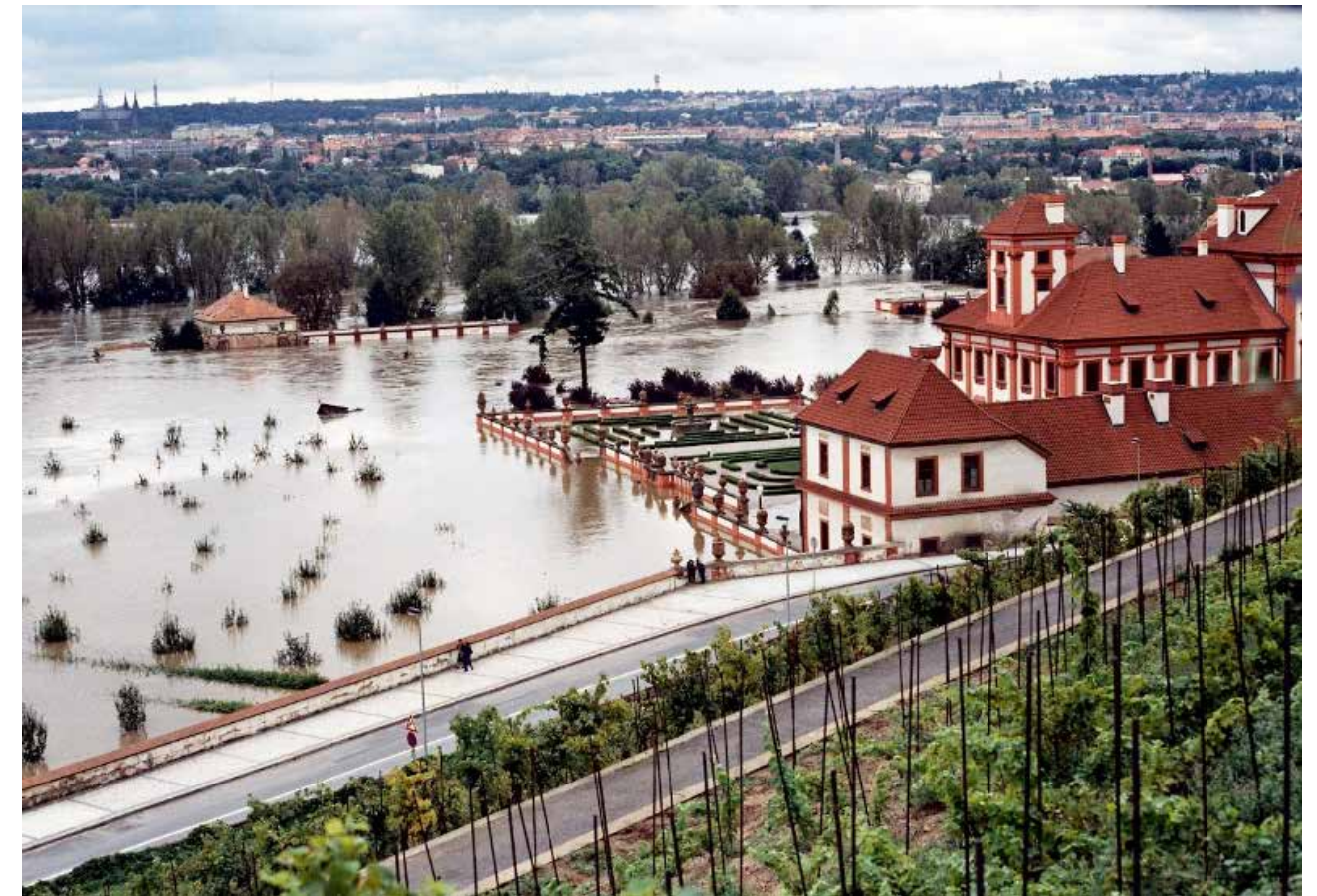
Fig. 1 Flooded garden of Troja Château. © Archives of the Troja Municipal District
