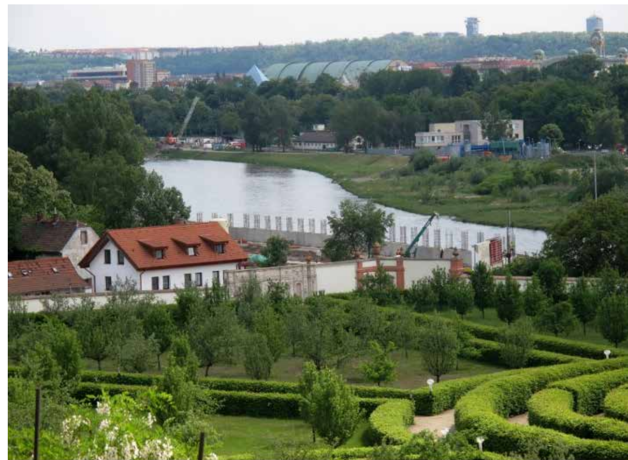
Fig. 3 A view of the construction of the rampart with pillars for the temporary wall and the connection to the Troja Château garden. © T. Drdáký
