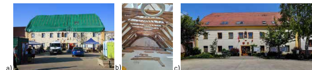
Fig. 5 - Town Hall: the Town Hall building after the intervention (a), the reconstruction of the Baroque roof (b), the renovated Town Hall building (c). Source: https://www.mnves.cz/projekty/obnova-budov-po-tornadu-obnova-radnice/
