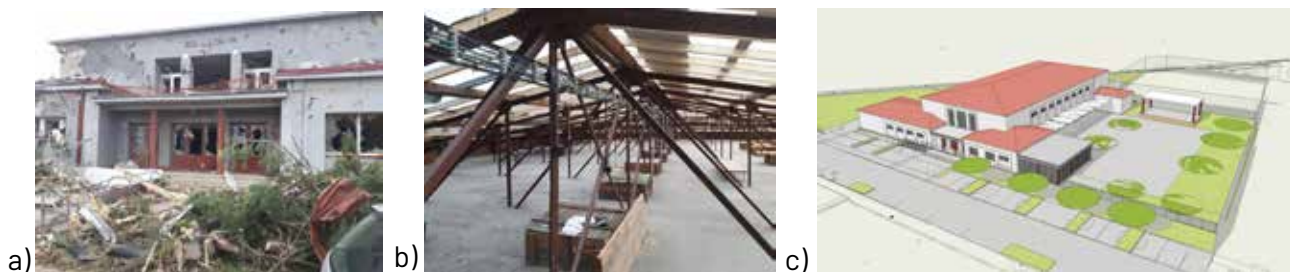
Fig. 8 Sokol hall: damage after the hit (a), reconstruction of the roof truss (b), visualization of the reconstruction design (c). Source: https://www.mnves.cz/projekty/rekonstrukce-sokolovny/
