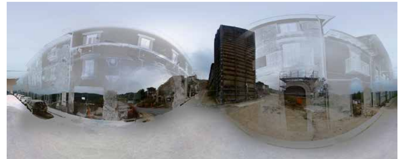
Fig. 4 360° panorama showing the overlay of the pre-earthquake condition with the current state. Source: Authors
