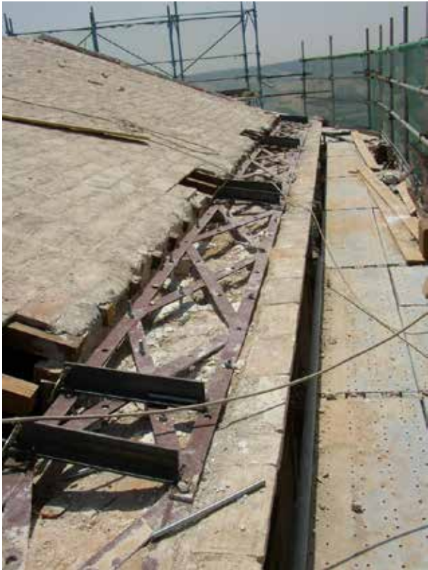
Fig. 5 Insertion of steel curbs in a historic masonry construction.
