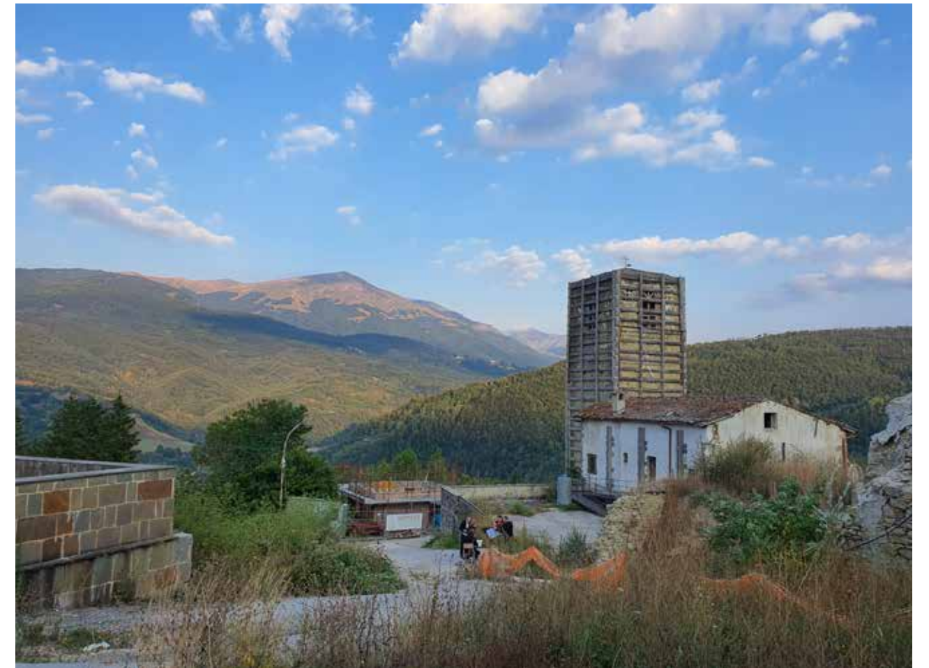
Fig. 1 The tower of Accumoli – a symbol of its identity – wrapped in reinforcing structure which helped it to survive the second earthquake in 2017. (Author)
