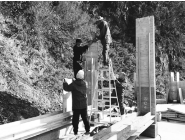
Fig. 2a Participatory construction of the Maeamihama Veneer House. (image by Hiroto Kobayashi).
