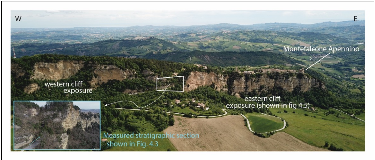
Figure 4.2. Aerial overview of the cliff-side exposures beneath the village of Montefalcone.
