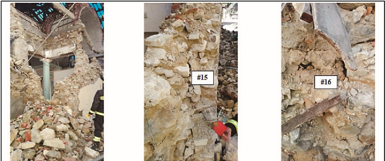
Fig. 3. Mortar sampling campaign in Pretare – St. Rocco Church (Arquata del Tronto)
