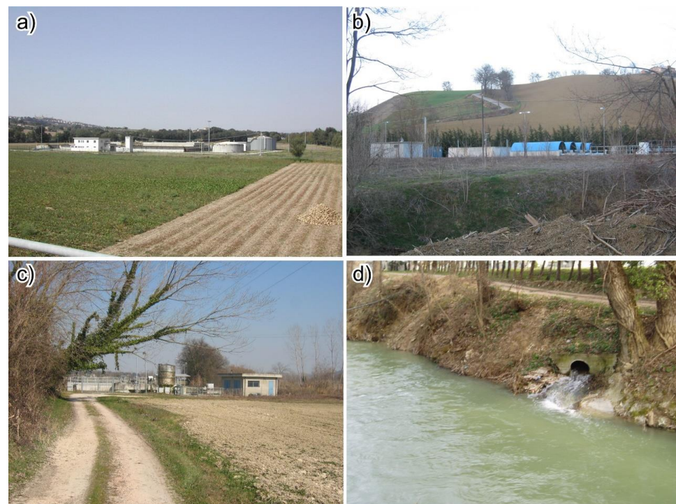
Figure 3. (a–c) the wastewater treatment plants of Tolentino, Camerino and Servigliano, respectively; (d) typical waste collector present along the riverbeds in correspondence of the main plants.
