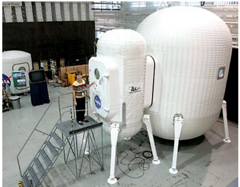
Fig. 52 - A demo of an inflatable structure sits at NASA's Langley Research Center in Virginia, US. A similar structure may be sent to Antarctica in 2008 to see how it weathers the extreme conditions there (Image: NASA/ Jeff Caplan)
