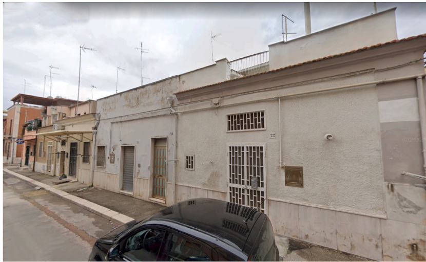
Fig. 10. Photo of the real row masonry aggregate used for purpose of validation.
