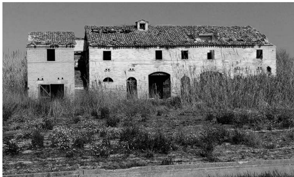
Figure 15. Building addition in the Tronto valley. (Source: Sara Cipolletti, 2022).
