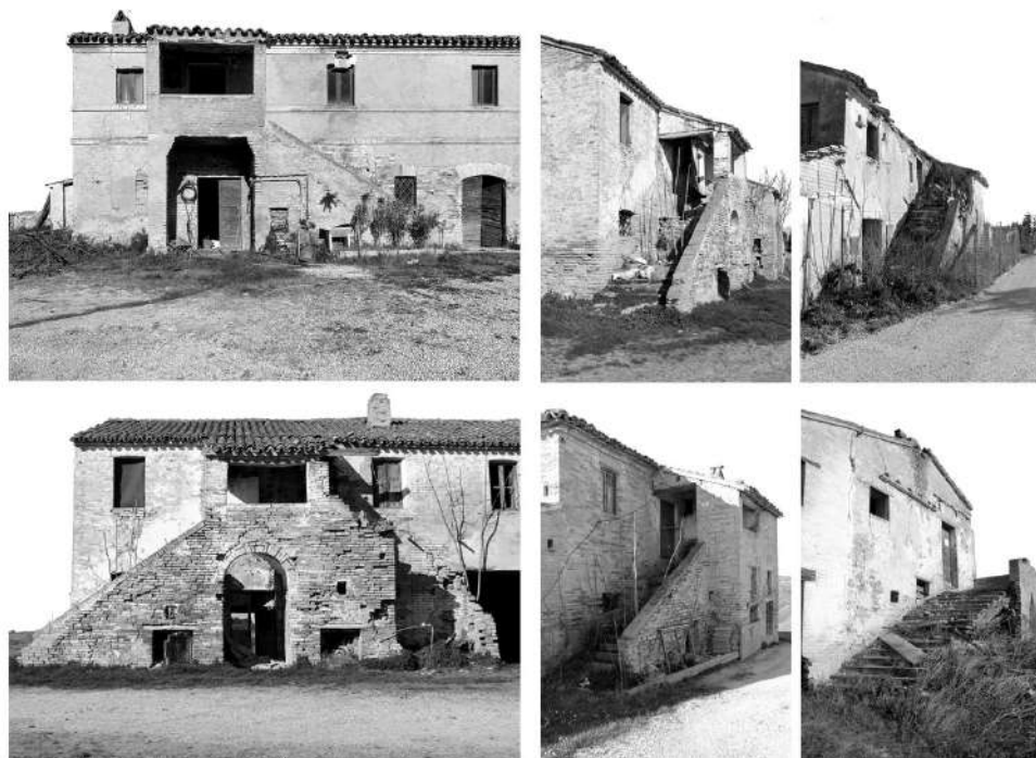
Figure 11. Variations of the external staircase in the hilly territory of Tronto and Tesino Valleys. (Source: [14]).
