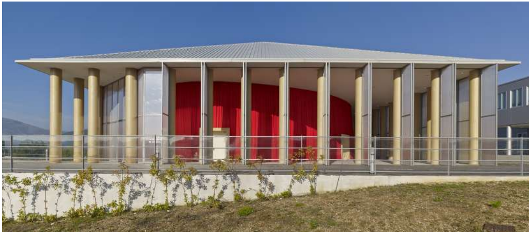
Figure 41 Temporary Concert Hall designed by Shigeru Ban Architects, 2011
