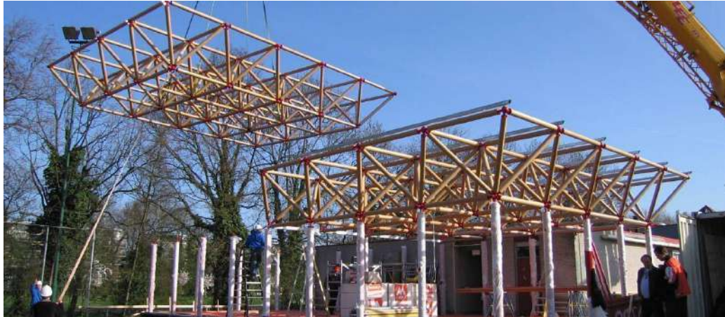
Figure 17 Picture taken during the positioning of the roofing structure
