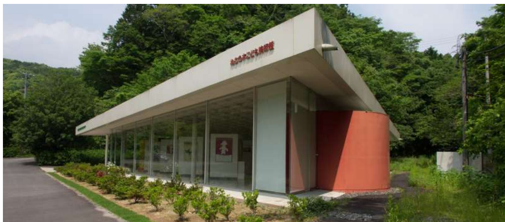
Figure 11 Nemunoki Children's Art Museum designed by Shigeru Ban Architects, 1999
