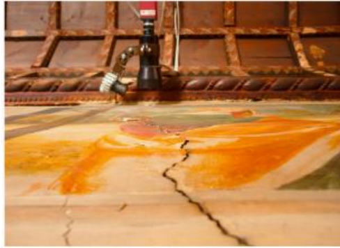
Figure 18: Conegliano Cathedral – crack survey with contactless sensor [Lorenzoni et al. 2015] [44]
