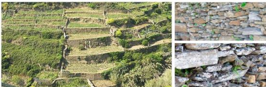
Figure 5.3 Left: the cultivated terraces in Cinque Terre; right: drywall maintenance is a significant factor in managing hydrological risk.
