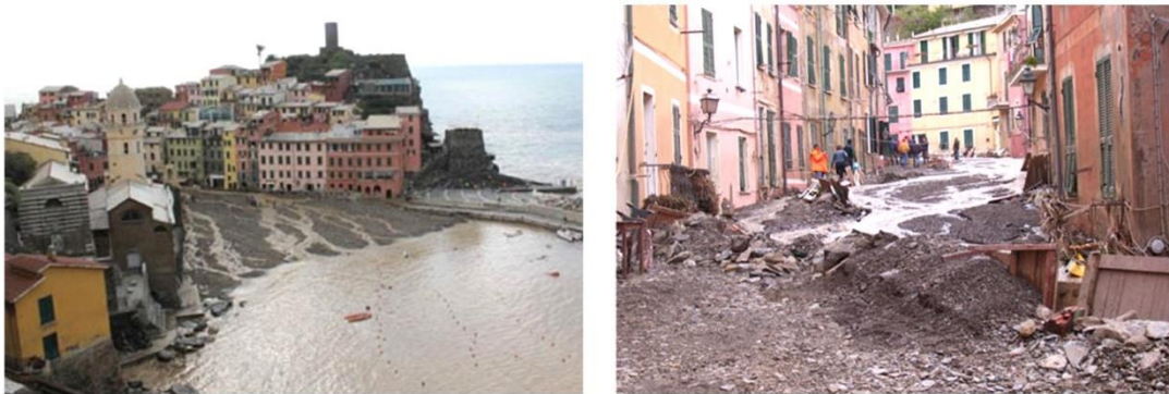
Figure 5.4 The flood of October 25, 2011, in Vernazza caused run-off, landslides, and the collapse of the terraced slopes (Brandolini, 2017).
