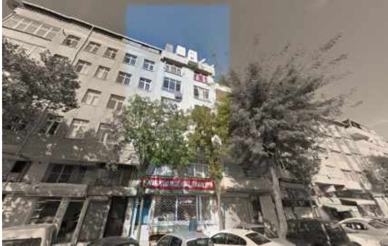
Figure 13 - Bad practice for urban renewal.
