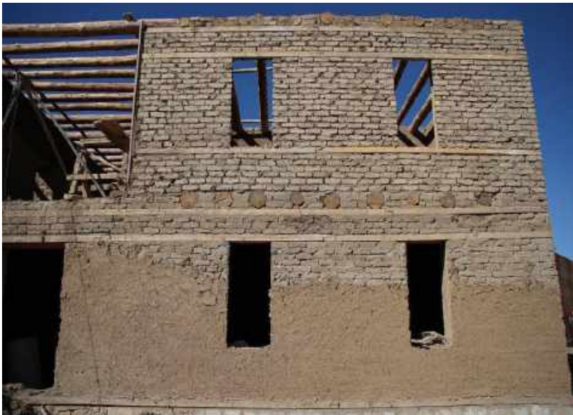
Figure 3 - Adobe house with anti-seismic presides
