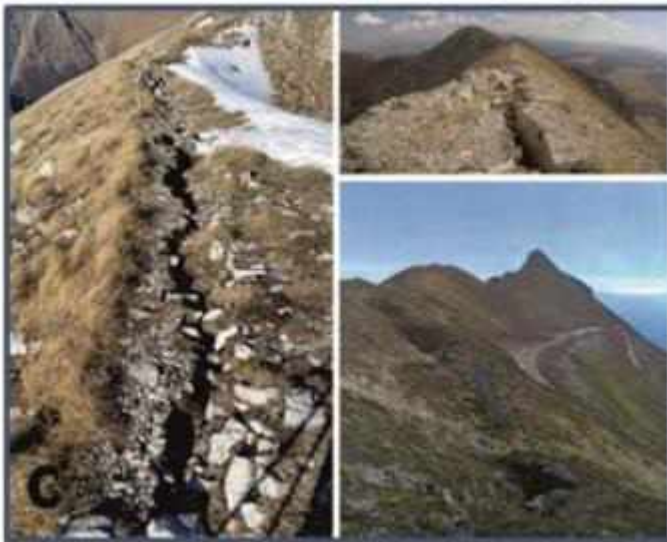
Figure 5 - Fracturing and ground cracks.
