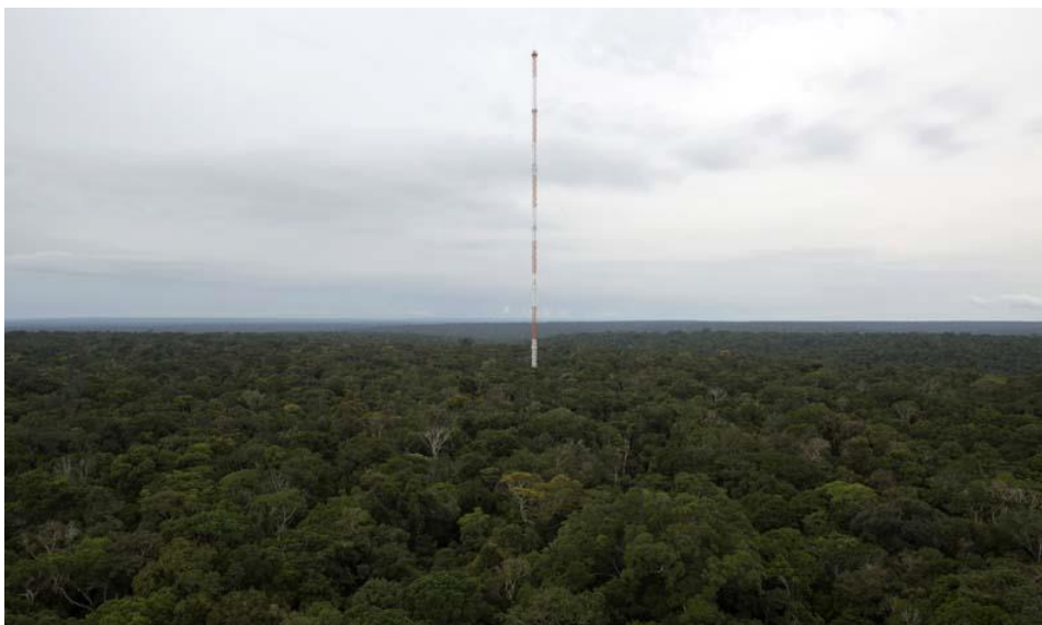
Figure 4.2: ATTO tower 325 m tall, used to support sampling instruments.
