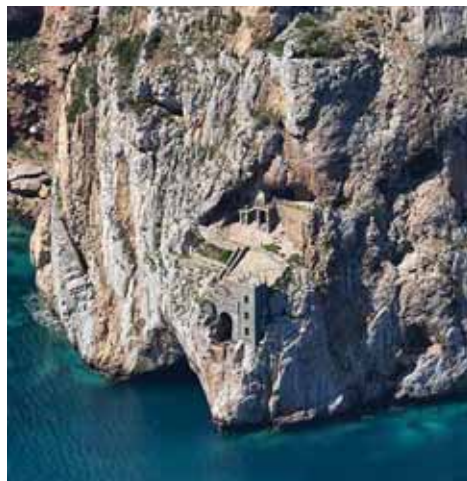
Fig. 08 : The system of terraces that connect the mouths overlooking the sea, of the loading and unloading tunnels, photo by Gianni Alvito, Archivio Parco Geominerario Sardegna
